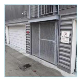
Pedestrian gate appears to be deteriorating at a rate typical of its age. Complete touch up paint, maintenance and repairs (paid from Operating Account) to help extend useful life cycles. These types of metal gates are typically durable, however, we recommend setting aside funding for regular intervals of replacement due to constant usage, wear exposure to the elements.
