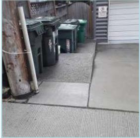
Repair contingency for the concrete surfaces on site. Amount and cycle to be reviewed annually. No widespread damage or deterioration noted at time of site visit. We recommend repairing trip hazards immediately to limit liability.
