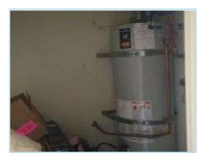
Hot water heaters/tanks are assumed to be in operation condition. We recommend budgeting for replacement at the timeframe indicated and before total failure which can lead to damage if a leak develops. Annual inspections by a qualified professional suggested.
