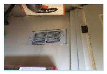
Wall heater are reportedly in functional condition. We recommend funding for replacement of this component at the timeframe indicated as these types of wall heaters will typically fail at roughly the timeframe estimated.
