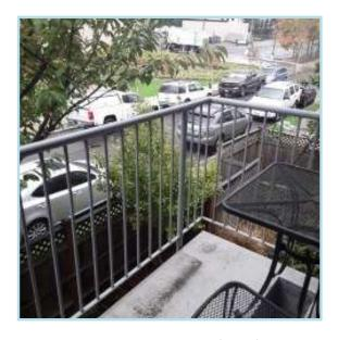
These metal rails should be inspected and monitored rails for safety, touch up paint annually & repair as needed from operating budget.
