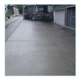
This component is for the replacement of the concrete driveway surfaces which was reportedly replaced in 2016. No widespread damage or deterioration noted at time of site visit. We recommend repairing trip hazards immediately to limit liability.
