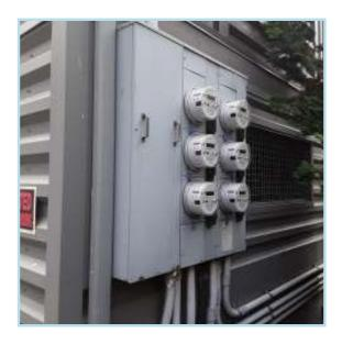
Electrical meter sockets appear to be deteriorating at a rate typical of their age. We recommend that a qualified professional be consulted to evaluate these systems and determine the current condition and repair/modernization needs.
