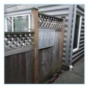
Appears to be deteriorating at a rate typical of its age based on our visual inspection of this component. As routine maintenance, inspect regularly, clean by wiping down for appearance, change lock cylinders, lubricate hinges and repair as needed from operating budget. Best to plan for total replacement at roughly the time frame indicated due to constant usage and wear over time.
