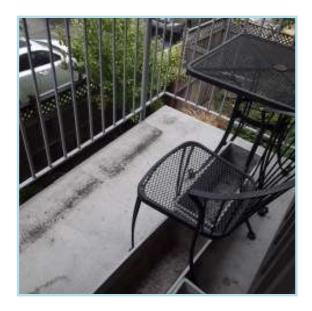
Resurfacing & refurbishing the decks involves removing the waterproof deck system and installing a new system, making any necessary repairs to the beams and sheathing. Local repairs to the deck sheathing and supports beams would also be included in this project as-needed and have been considered in this cost estimate.
