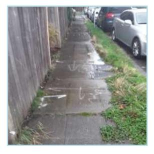
Repair contingency for the concrete public sidewalks. Amount and cycle to be reviewed annually. Several trip hazards and cracks noted during the site inspection. We recommend repairing trip hazards immediately to limit liability.
