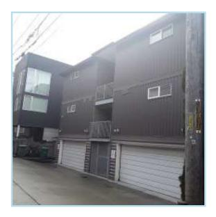
Garage doors appear to be deteriorating at a rate typical of their age. If not damaged or abused garage doors will last the estimated useful life indicated; repair as needed from operating funds. Clean and paint along with other exterior building surfaces. Best to plan for eventual replacement due to constant usage and wear over time.
