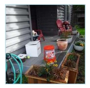
Composite decks appear to be deteriorating at a rate typical of their age. As part of ongoing maintenance program, inspect regularly for any damage/deterioration and repair promptly as needed from operating budget. Clean regularly for appearance, maximum design life and to ensure adequate footing. We recommend budgeting for full replacement of these exposed decks due to constant exposure to the elements.
