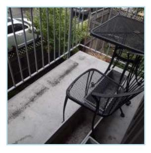
This membrane surface with non-skid material needs to be top coated periodically for waterproof integrity, protection of surrounding structure, appearance and non-skid properties. As routine maintenance, we strongly suggest annual professional inspections, with cleaning and repair as needed. Clean with mild solution such as TSP; bleach can be added if mold/mildew becomes a problem. Plan for regular intervals of professional maintenance top coating at the interval indicated.
