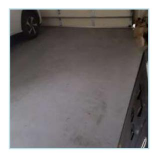
The garage coating appears to be deteriorating at a rate typical of its age. As routine maintenance, inspect regularly and touch up/repair locally as needed using operating funds. Typical coating cycles for these surfaces are between four to six years depending upon surface preparation, material quality, application methods, pedestrian traffic volume and site & weather conditions.
