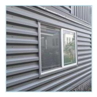
The vinyl windows appear to be deteriorating at a rate typical of their age. No reported problems such as water intrusion. As routine maintenance, we recommend regular professional inspections and prompt repair as needed to ensure building waterproofing and help prevent structural damage. If properly installed without defect, plan to replace at roughly the time frame indicated.
